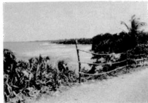
Fig. 11. A temporary bamboo guard rail in the parish of Portland.
